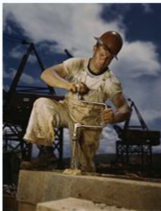
Fig. Carpenter using a crank-powered brace to drill a hole.
